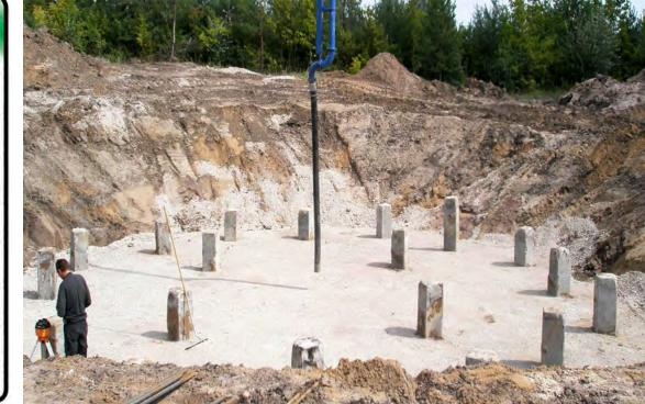
Landfills, mining legacy landscapes and abandoned industrial sites are generally inexpensive and exposed locations that are suitable for wind turbine development. Since the soils of these sites are usually of low bearing capacity down to greater depths, their development requires innovative solutions in foundation planning.
