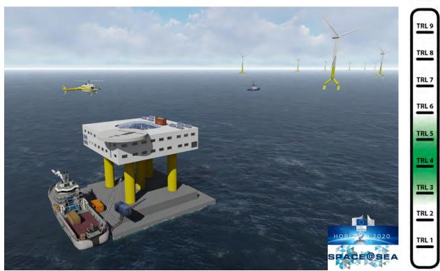
The aim of Space@Sea is to develop sustainable artificial islands that can be assembled in modules. The project aims to develop low-cost, floating platforms that can be used off the coast as logistics, housing, energy and/or aquaculture bases. The background for the project is, among other things, the ever-increasing population and limited land area worldwide. Due to the increasing demand for renewable energy and food, new forms of residential and logistics centers are required.
