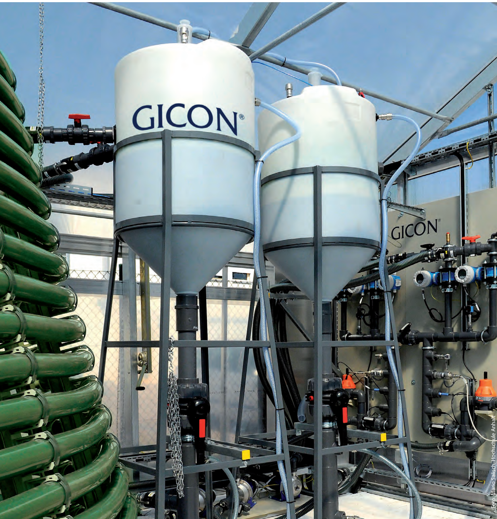
Mixing tank at the microalgae photobioreactor plant, Anhalt University of Applied Sciences, Köthen (Germany)
