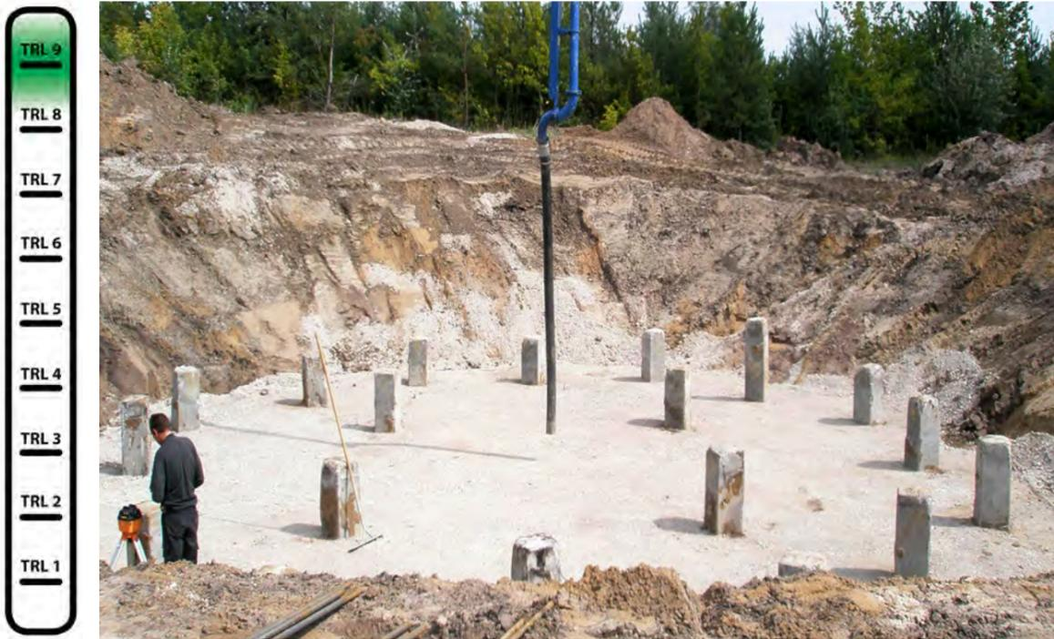
Landfills, mining legacy landscapes and abandoned industrial sites are generally inexpensive and exposed locations that are suitable for wind turbine development. Since the soils of these sites are usually of low bearing capacity down to greater depths, their development requires innovative solutions in foundation planning.
