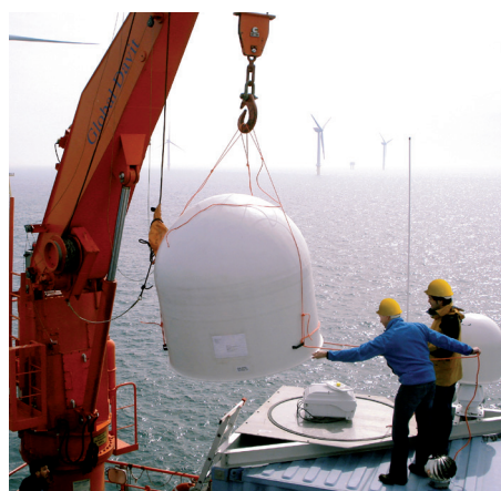
Installation of the GICON/IfaÖ radar
