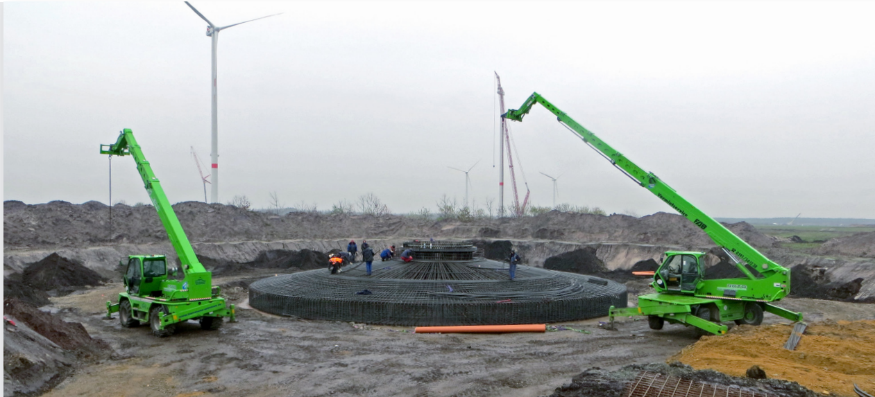
Installation of foundation reinforcement at the wind farm building site in Klettwitz
