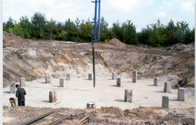
Installed driven piles at the wind farm in Cottbus Nord
