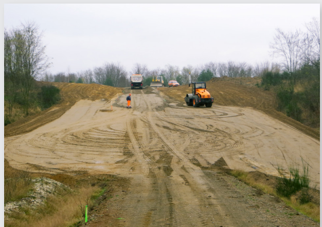
Road construction – flattening out the entry into a depression
