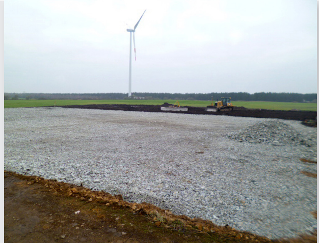
Creation of a crane erection site
